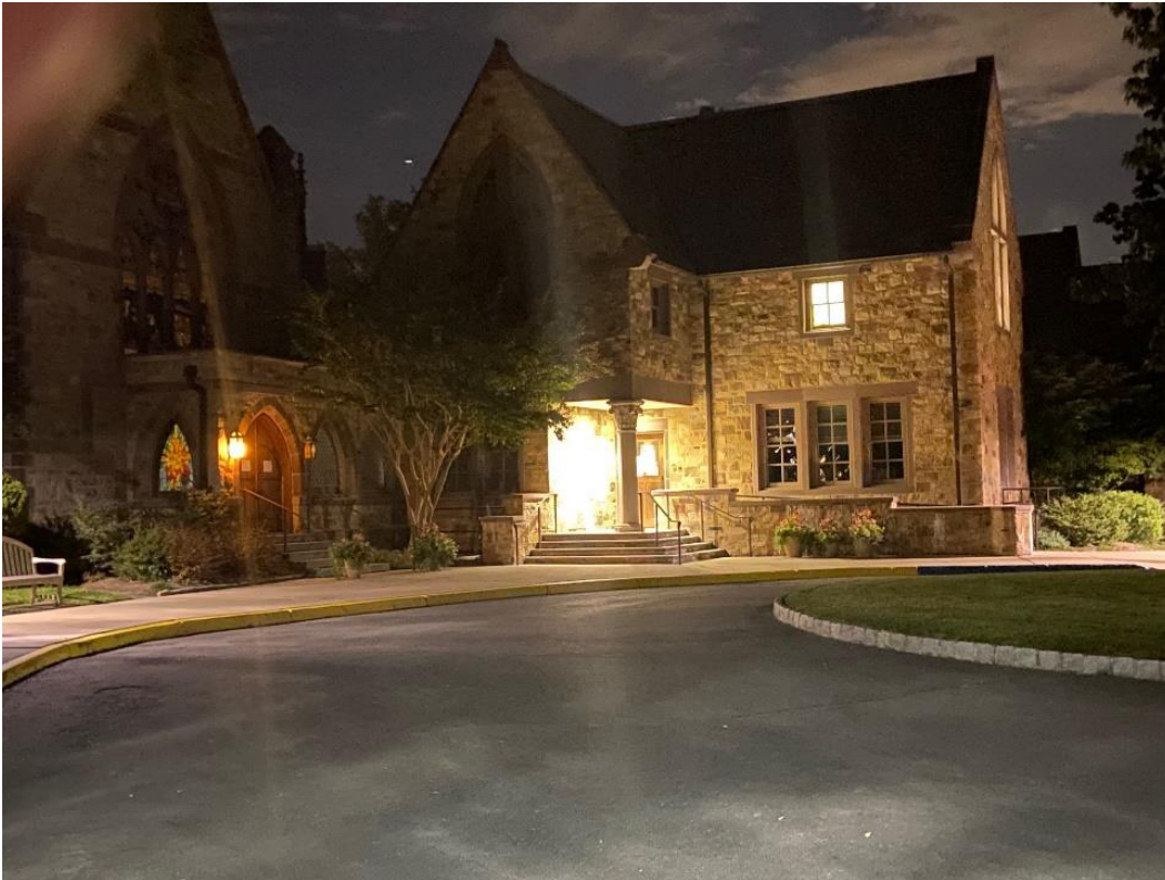
This view is the door (the one that is brightly lit, straight ahead) for the meeting entrance
